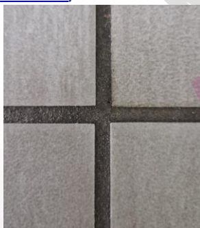
Joints avant application
